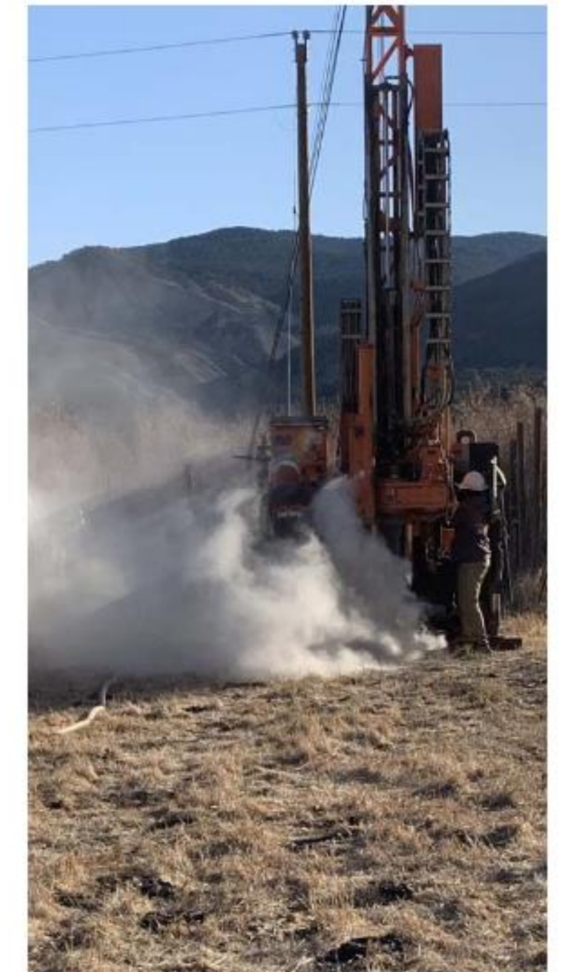
Dry soil for the first 35 ft of drilling at TW-1
